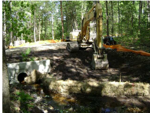
5/29/08 – Level Spreader Construction
