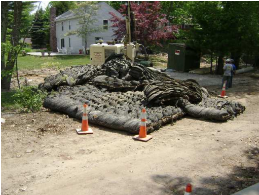
5/27/08 – Placing Blasting Mats
