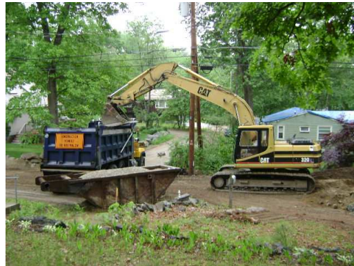
6/4/08 – Drainage Pipe Installation
