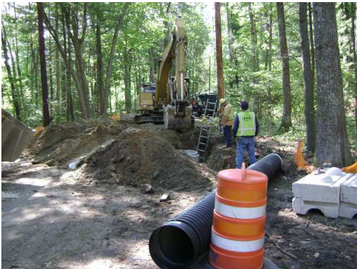
6/2/08 – Installation of a Catch Basin
